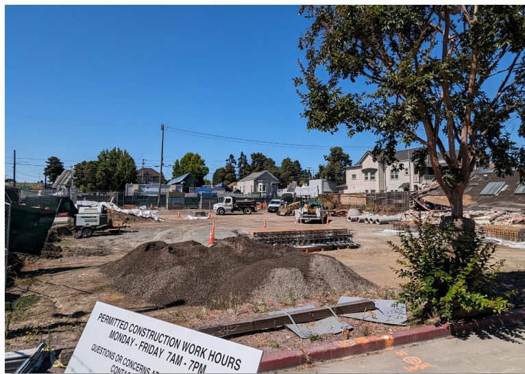
Cleanup and construction work in Oakland, CA
