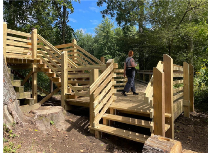
The completed observation deck
