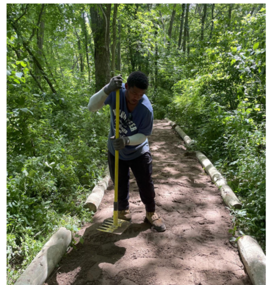
Groundwork Indy member tamping trail surface
