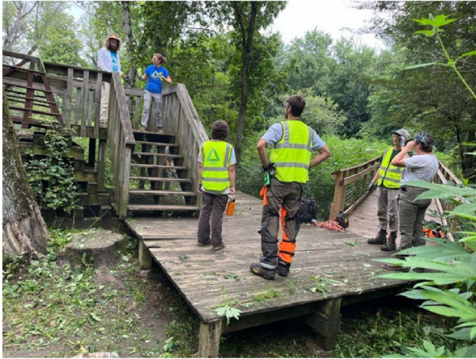
Inspecting the old deck before demolition
