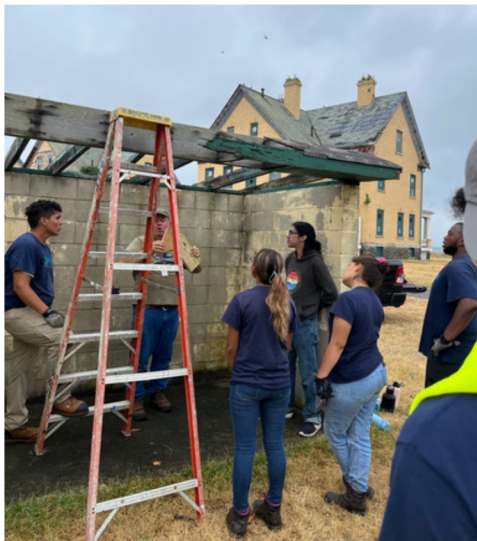
Groundwork Elizabeth discussing the roof
