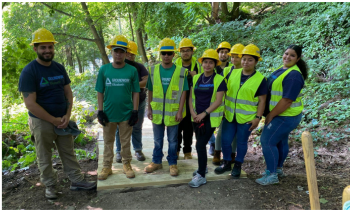
Groundwork Elizabeth with the finished staircase
