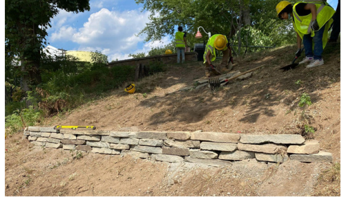
Final touches on the retaining wall
