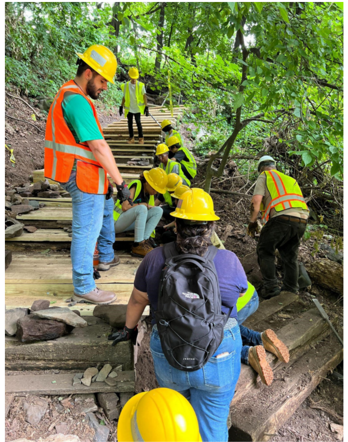
Groundwork Elizabeth replacing and improving the staircase
