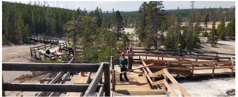
Groundwork RVA working on the boardwalk.
