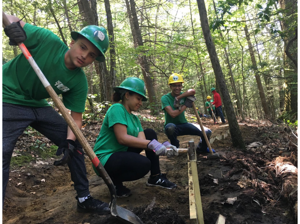
Youth from Groundwork Lawrence (MA) Green Team learn carpentry and conservation skills by building a retaining wall at the Deer Jump Reservation in Andover, MA. Photo: Groundwork Lawrence
